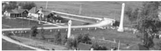
Two Range Towers
